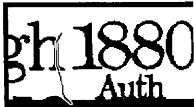
NEW —Crack found by Scott Hoppis.
